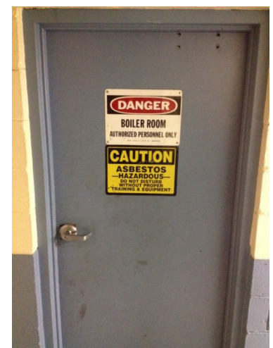
Figure 2: Asbestos Caution Sign Posted at Hilton Anchorage
